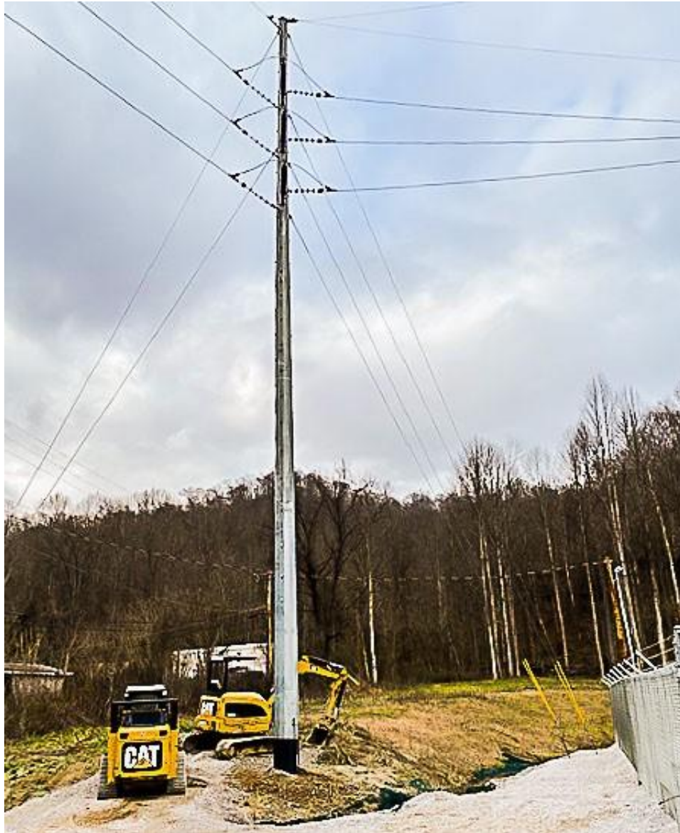
COMPARABLE EXISTING STRUCTURE PHOTOGRAPH
