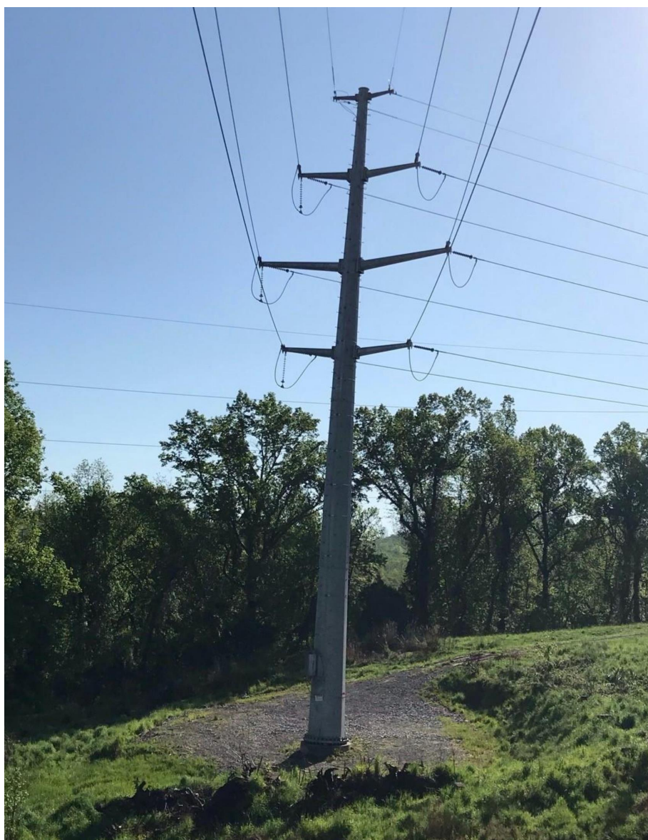
COMPARABLE STRUCTURE PHOTOGRAPH
