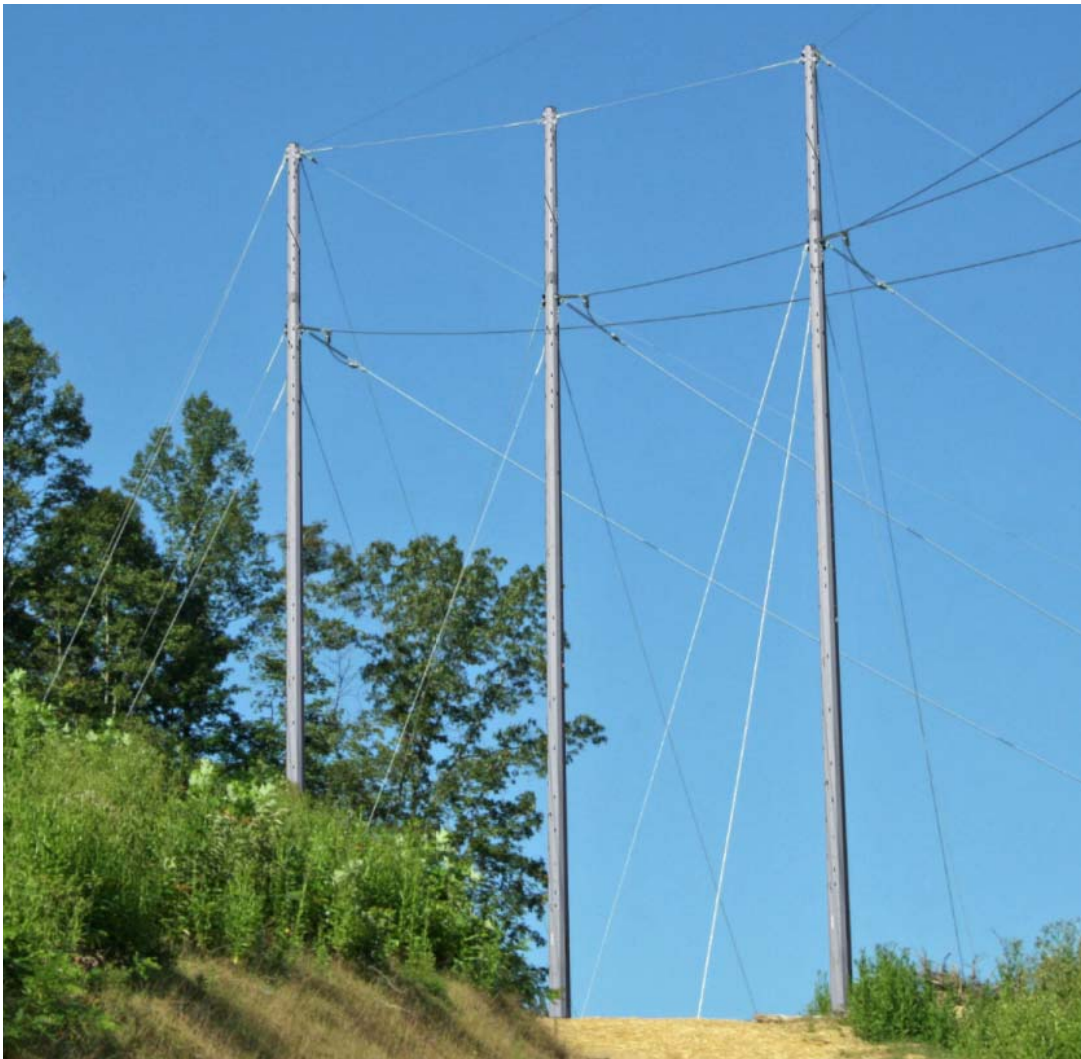
COMPARABLE EXISTING STRUCTURE PHOTOGRAPH
