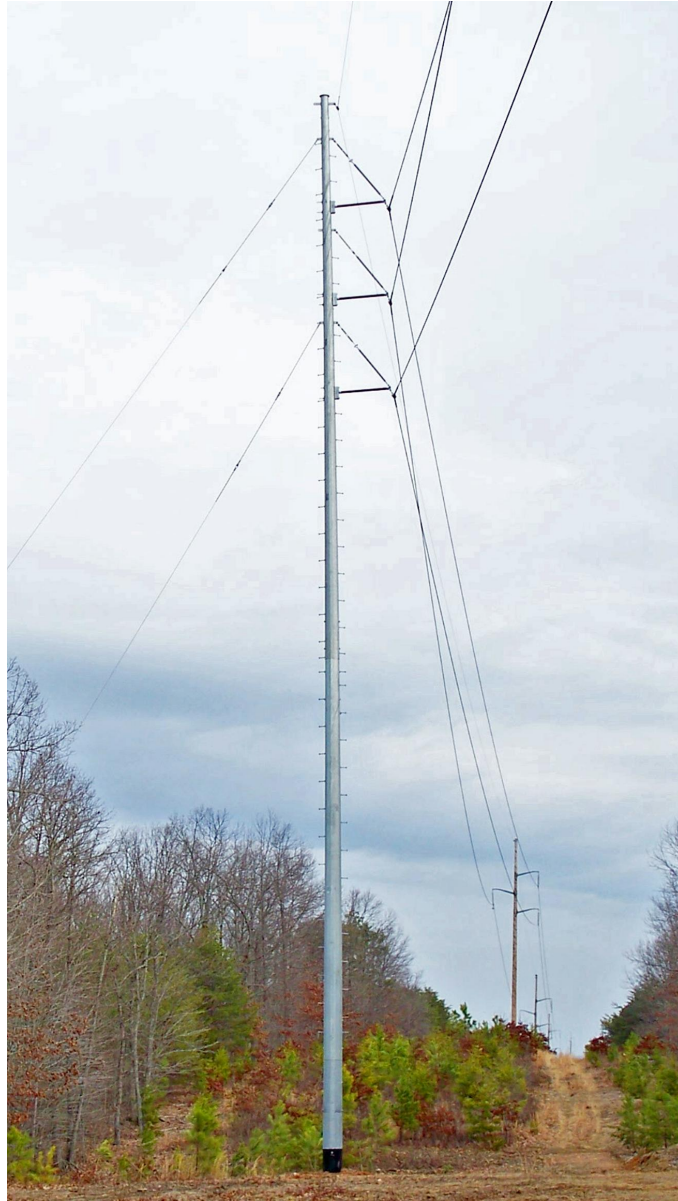
COMPARABLE EXISTING STRUCTURE PHOTOGRAPH
