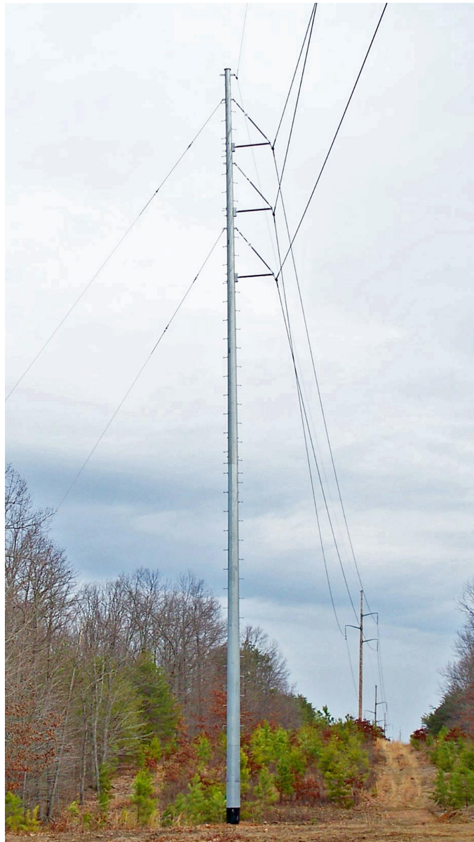
COMPARABLE EXISTING STRUCTURE PHOTOGRAPH
