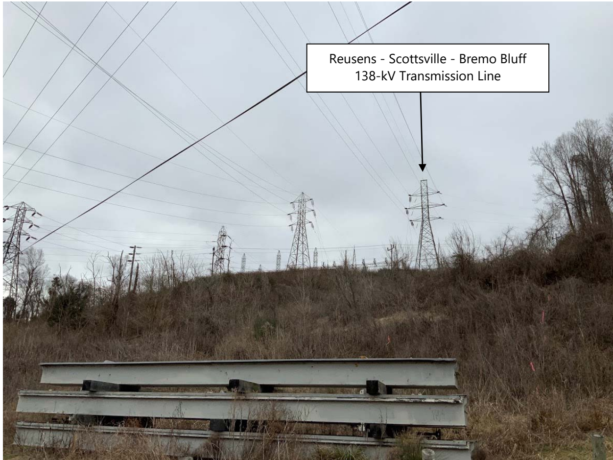
Existing Double Circuit Lattice Structures at the James River Crossing
