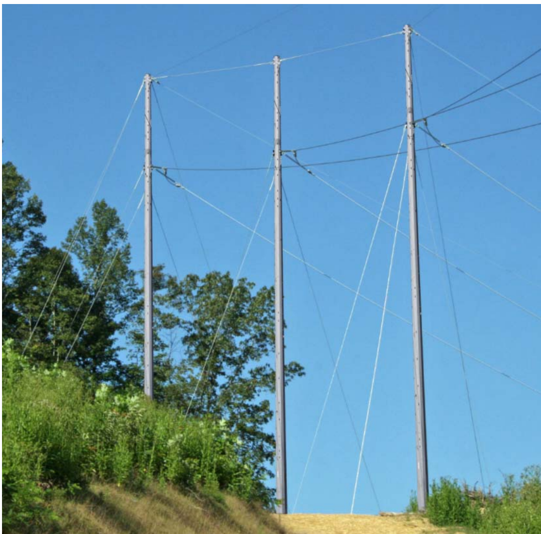
COMPARABLE EXISTING STRUCTURE PHOTOGRAPH
