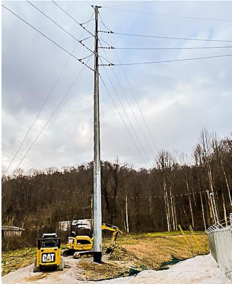
COMPARABLE EXISTING STRUCTURE PHOTOGRAPH
