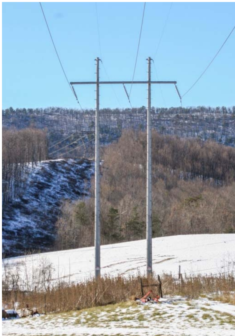
COMPARABLE EXISTING STRUCTURE PHOTOGRAPH
