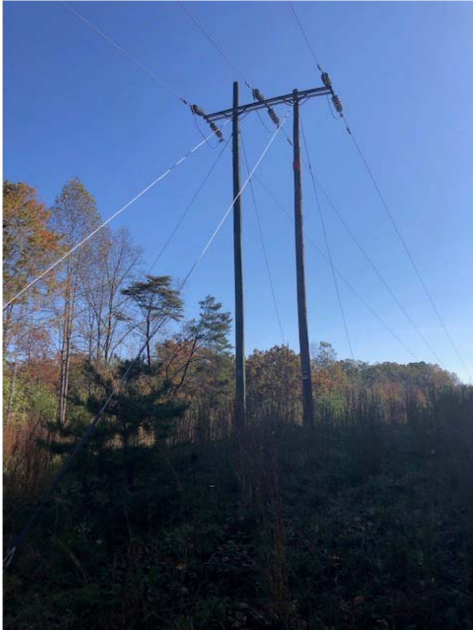
Existing H-Frame Structure with Guy-Wires
