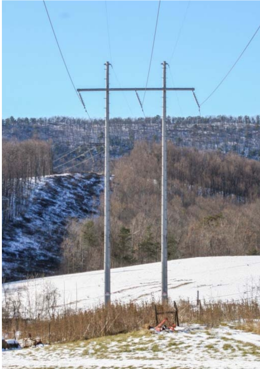
COMPARABLE EXISTING STRUCTURE PHOTOGRAPH
